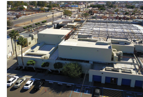
Mexicali, Mexico Back End Assembly and Test
